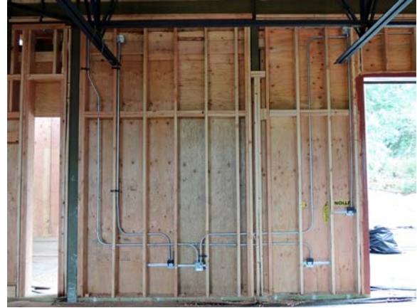
Electrical rough-in in progress at the upper level.
