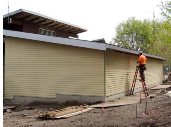
Siding installation in progress at the Storage Building.
