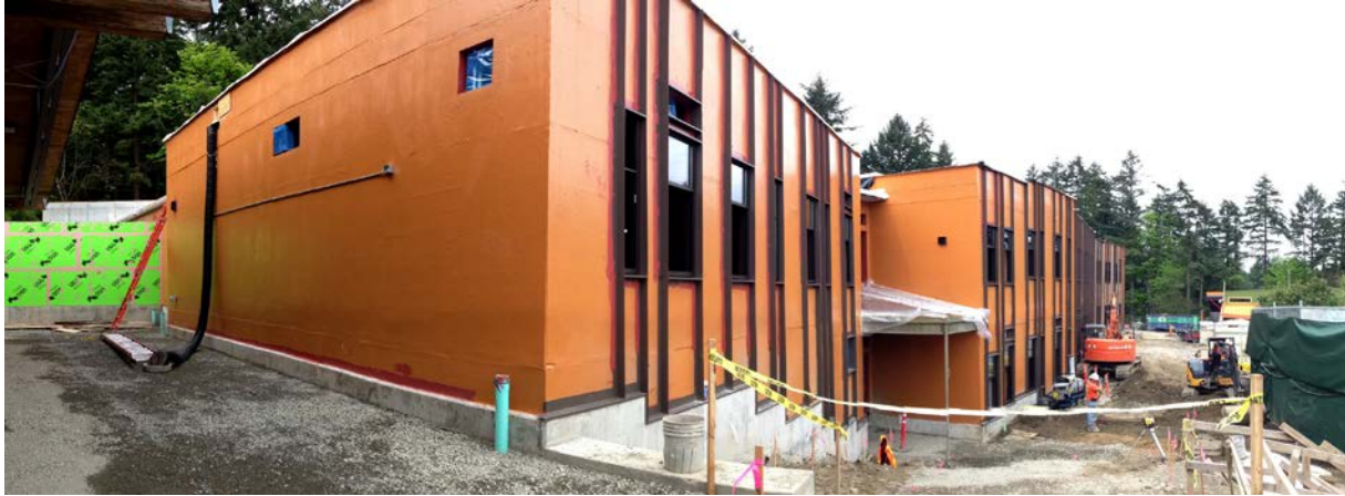
Overall construction progress looking northwest.
