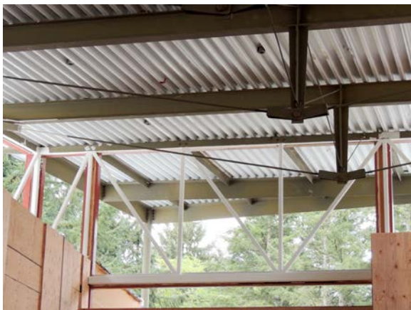
Priming structural steel in progress at the Clerestory.
